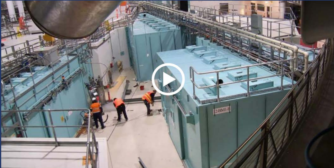
Construction of the MEX user cabins
