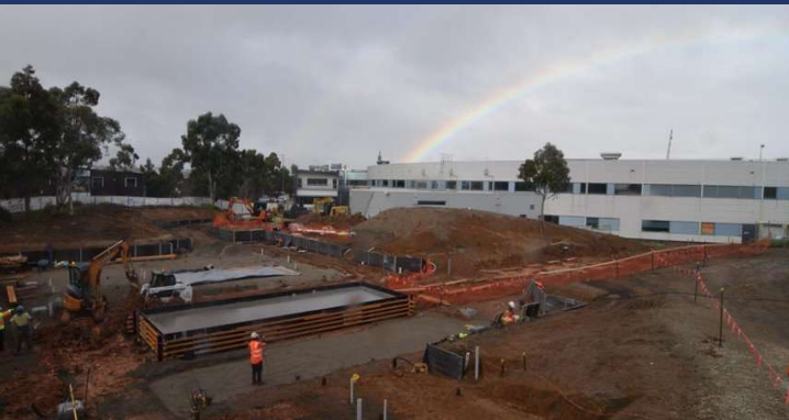
June 2023 pouring of the 900-mm thick endstation slab
