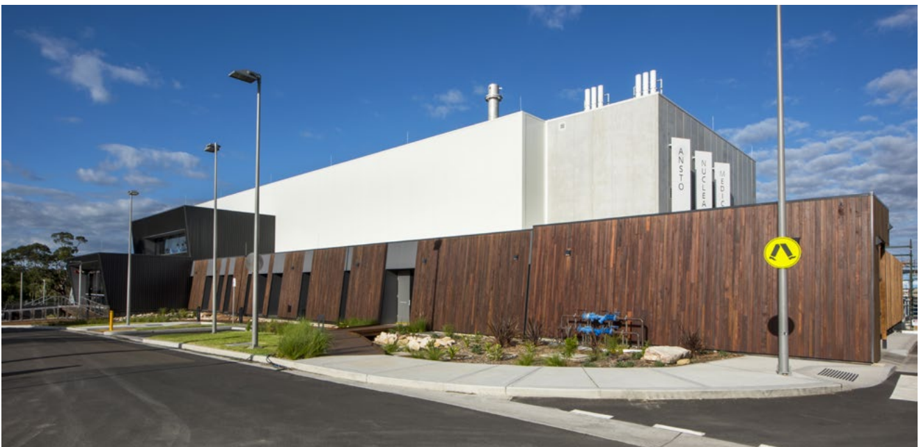
The ANSTO Mo-99 Manufacturing Facility.
