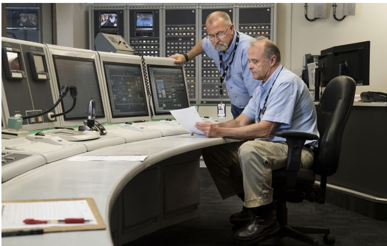
The OPAL reactor control room.
