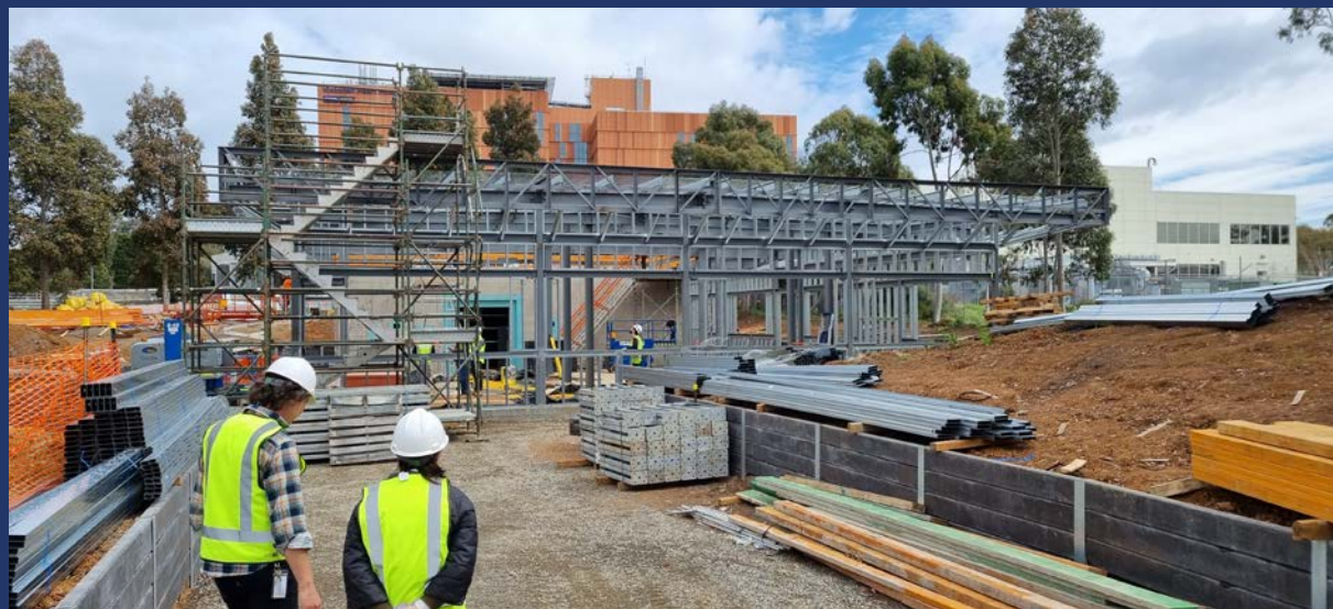
Nano satellite building progress
