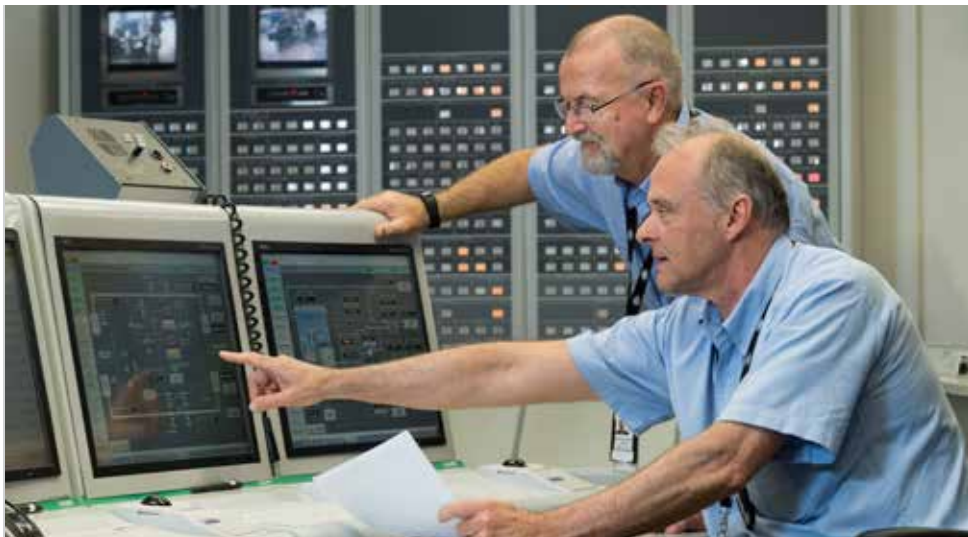
The upgrade to the Reactor Control and Monitoring System will extend the life of the control system by 10 to 15 years.
