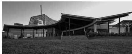
ANSTO's OPAL research reactor building.
