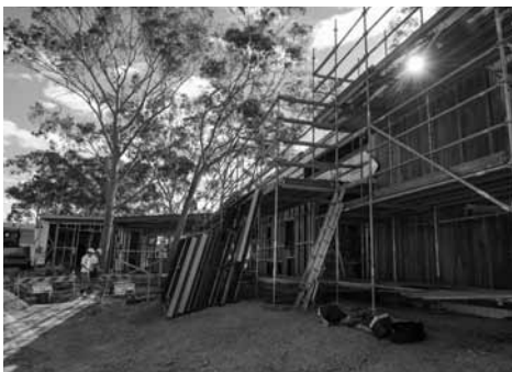
The ANSTO Childcare Centre under construction.
