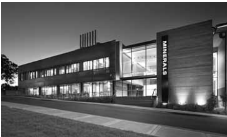
ANSTO Minerals main building.
