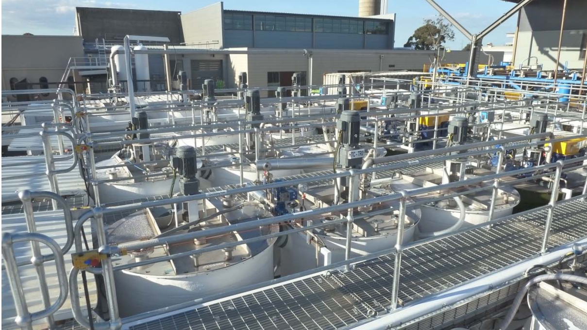
Figure C9 Brine processing demonstration plant at ANSTO – impurity removal circuit
