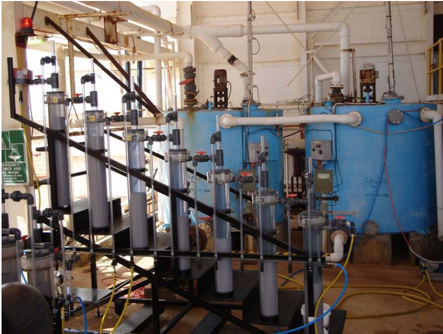
Figure A1 IX rig designed / built by ANSTO installed on site
